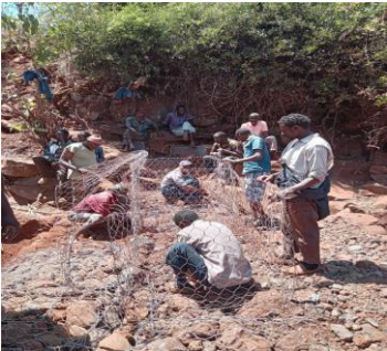
On –stream gabions check dam
